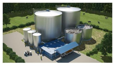
Image: A large dairy operation plans to use a multi-stage biological treatment plant to convert severely contaminated wastewater and liquid waste into biogas.
