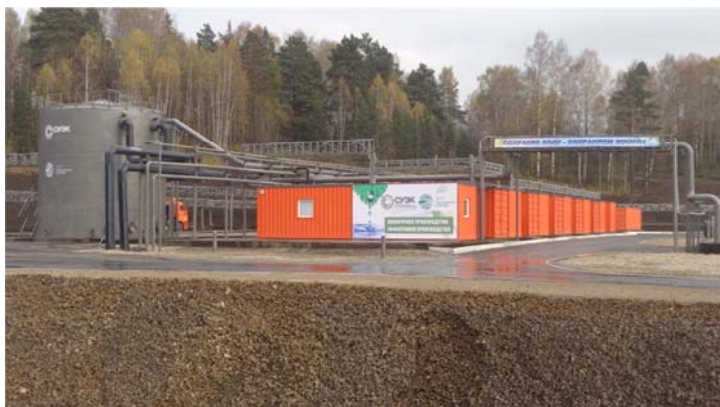
Image: Innovative modular wastewater treatment plant for the coal company SUEK-Kuzbass
