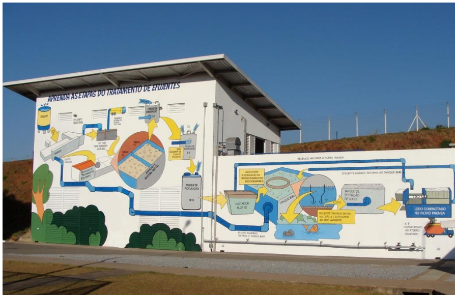
Wastewater treatment plant for wastewater from cosmetic production in Latin America
