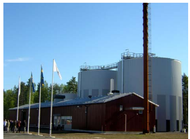
Full view of the biological wastewater treatment plant Biomar
