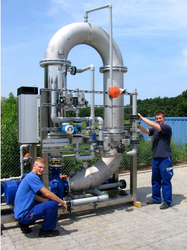
Fig-2: Example of an Envipur ultrafiltration installation's standardised module rack
