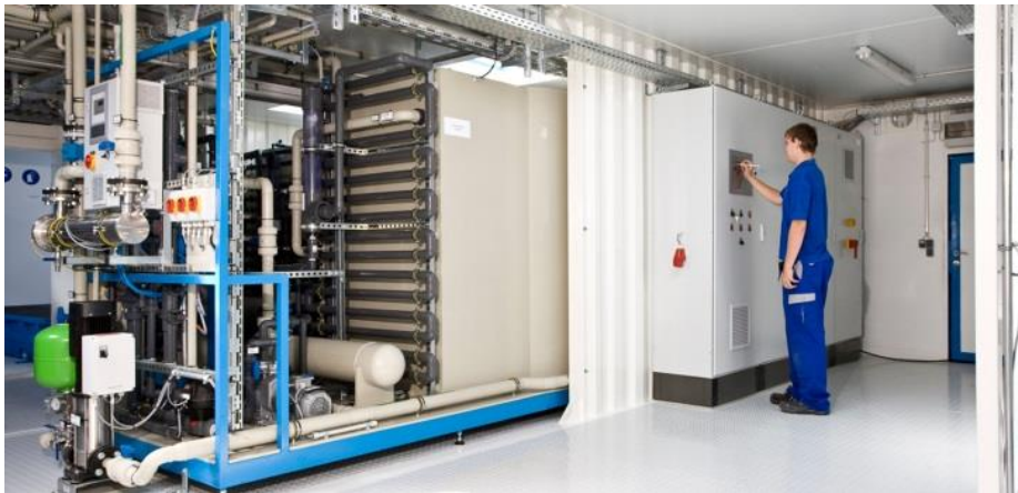
Image: Lugan ® flotation plant in a modular EnviModul system for the post treatment of dairy wastewater
