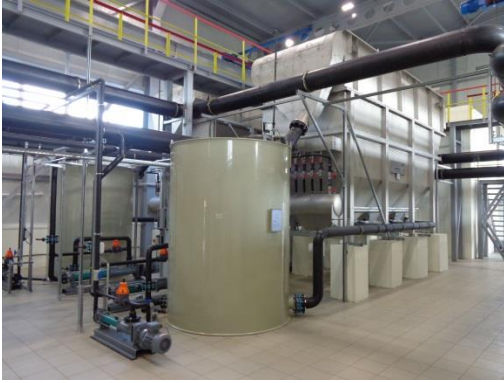
Image: Flomar® flotation plant with a capacity of 200 m 3 per hour, in use as a coalmine pit water treatment system
